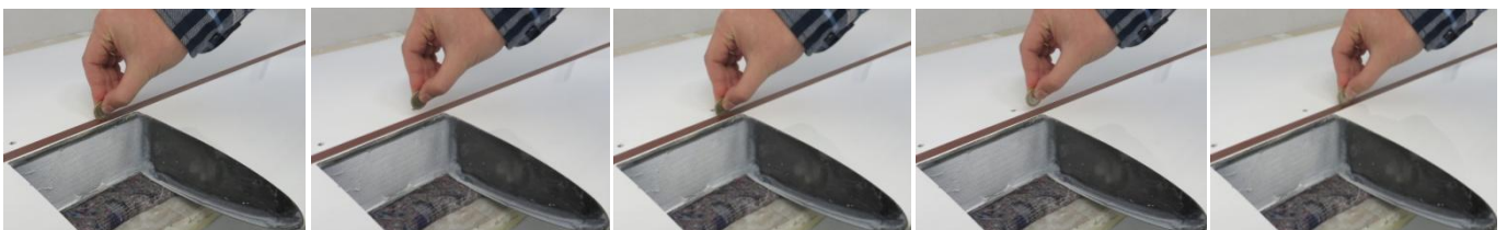
Fig. 3 – coin tap test along main wall position
